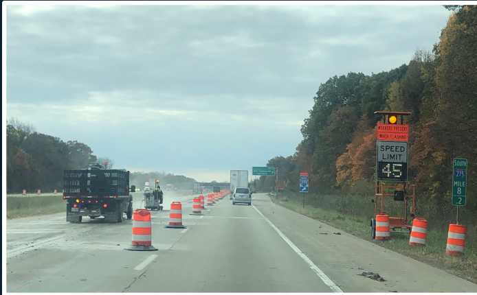
“Where Workers Present” Variable Speed Display
