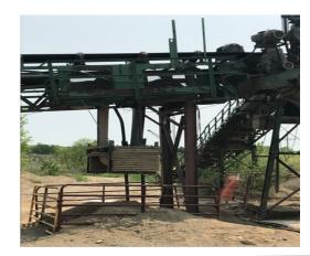
The area is difficult to properly guard leaving potential access to the take up pulley. When cleanup is required, in order to access the area, the cattle gates must be removed which can be awkward, buried by material, or difficult to move.
